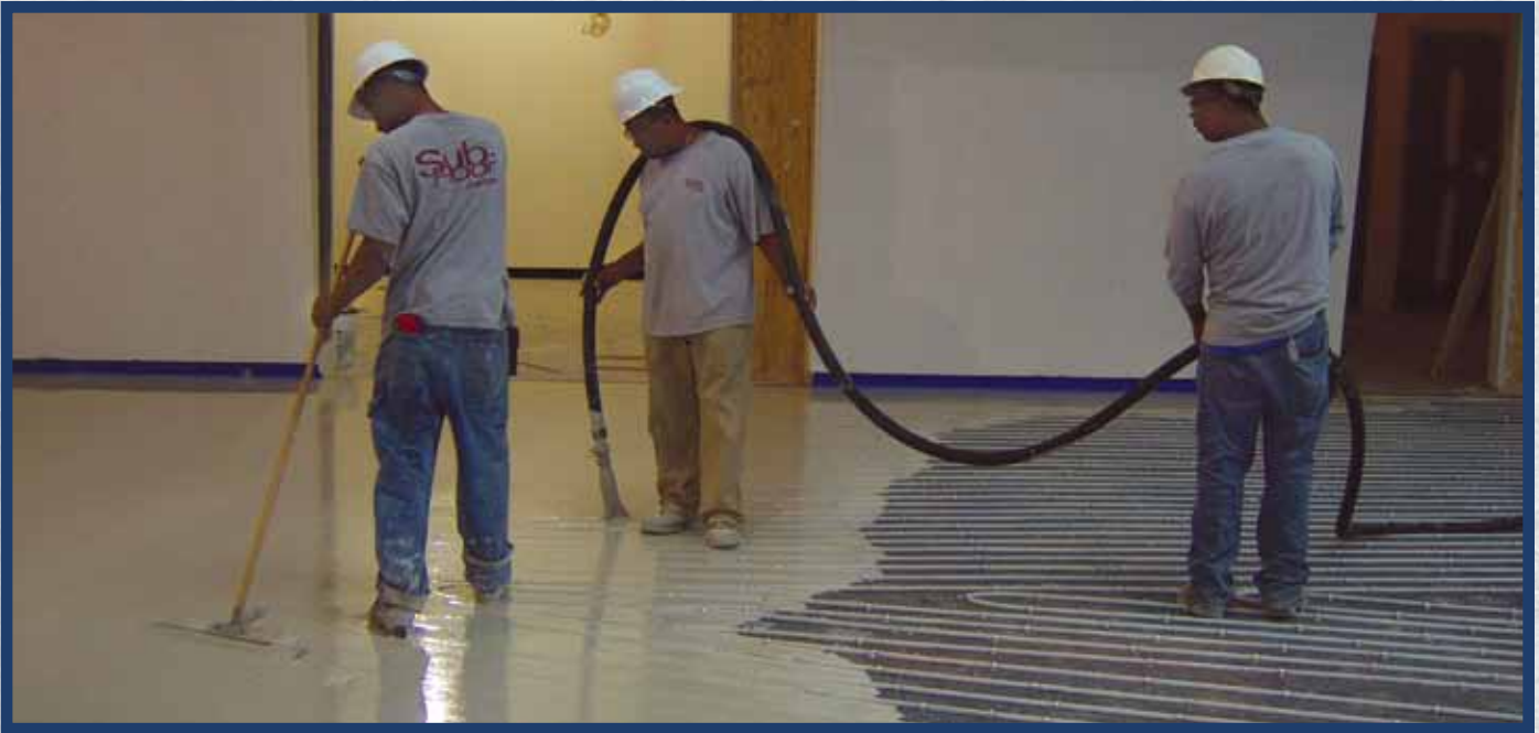
Sub-Floor Solutions offers a wide variety of products and services suitable for various applications, including polished concrete, stamped overlays, epoxy floor coatings, and, as seen here, heated floor systems, often used in high-end residential buildings.
